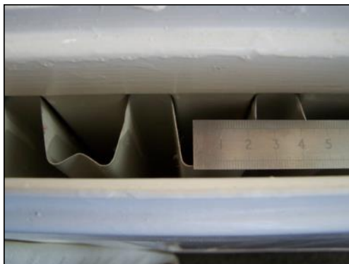
Photo. 5. A 'Type 21' domestic double panel domestic heating radiator.
